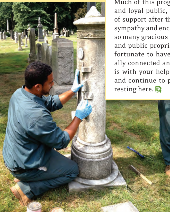
[Below] Green-Wood restoration team member Gustavo Padilla helps repair a 19th-century white marble monument.
