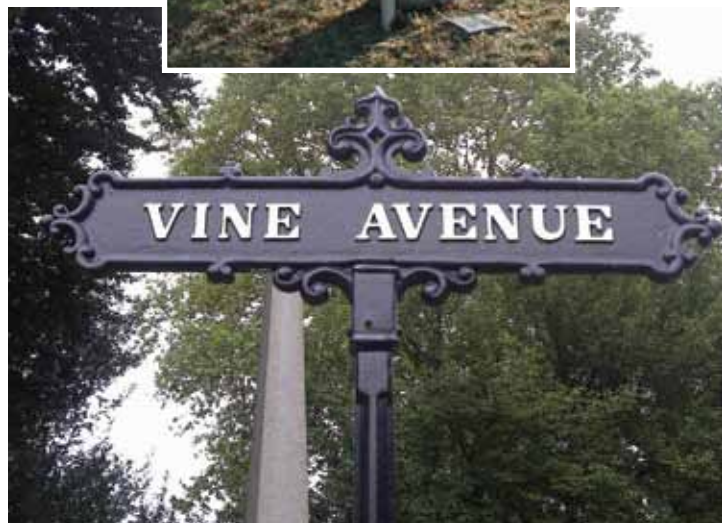
^ [top] A new batch of historically correct cast-iron signs arrives from the foundry; [inset] an example of an aluminum sign that will be replaced; [bottom] a newly installed cast-iron sign for Vine Avenue.
