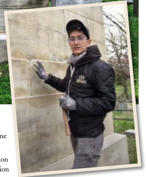
Neela explains mortar removal and replacement
