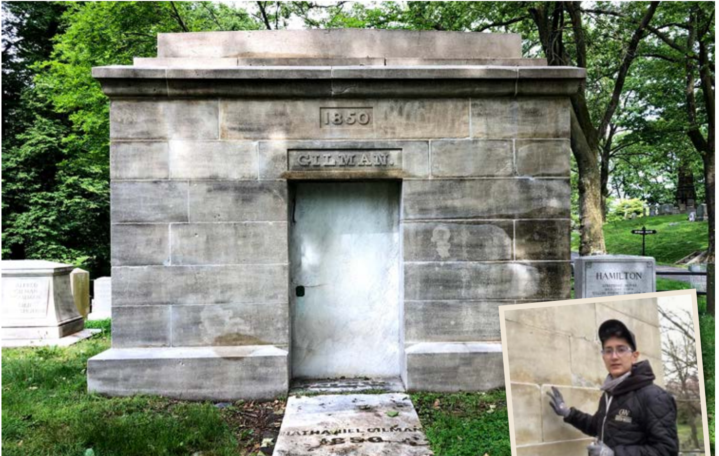
The newly repointed Gilman mausoleum
